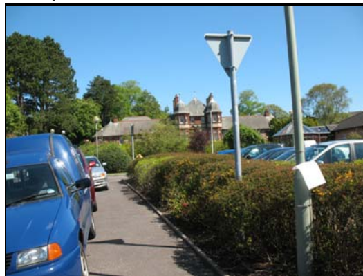
Photograph 2.1: Hospital access road to the west of the existing garden area
